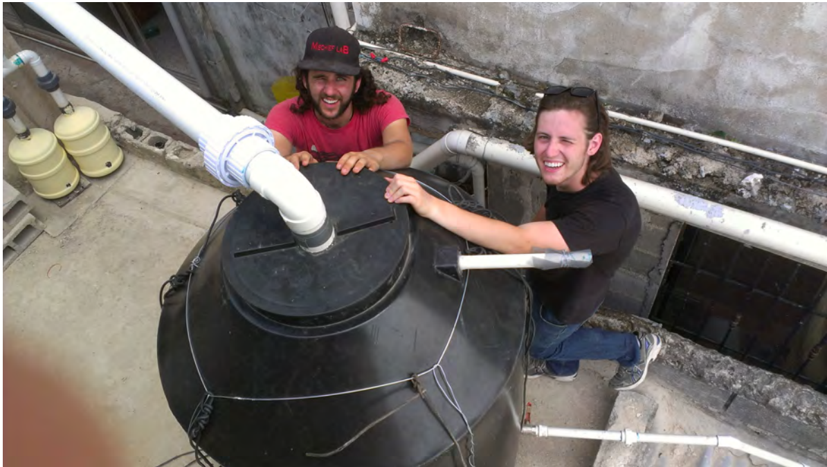
Figure 6.5: Community provided telephone wires and thick, galvanized wires were used to secure the storage tank to the cinderblocks on which the tank sat.
