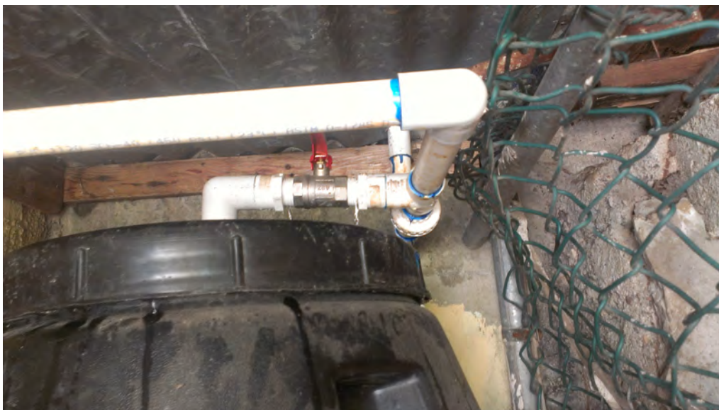
Figure 4.6: 1.5 inch pipe can be directed into the 35 gallon slow sand filter (black) or to a bypass (foreground).
