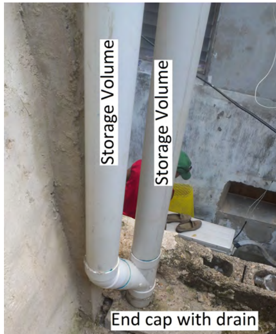
Figure 4.3: The first flush system was constructed entirely out of 3 inch PVC piping (storage volume) with an end cap at the bottom.
