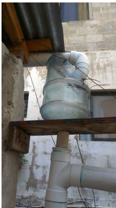
Figure 4.4: The Tee intersection directed the water to the 250 gallon storage tank.
