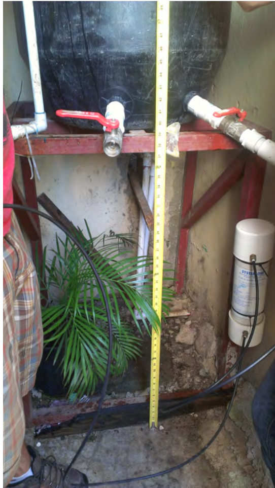
Figure 4.7: The filtered water was directed to a cartridge-style, silver-impregnated, activated carbon filter to further filter and disinfect the water.
