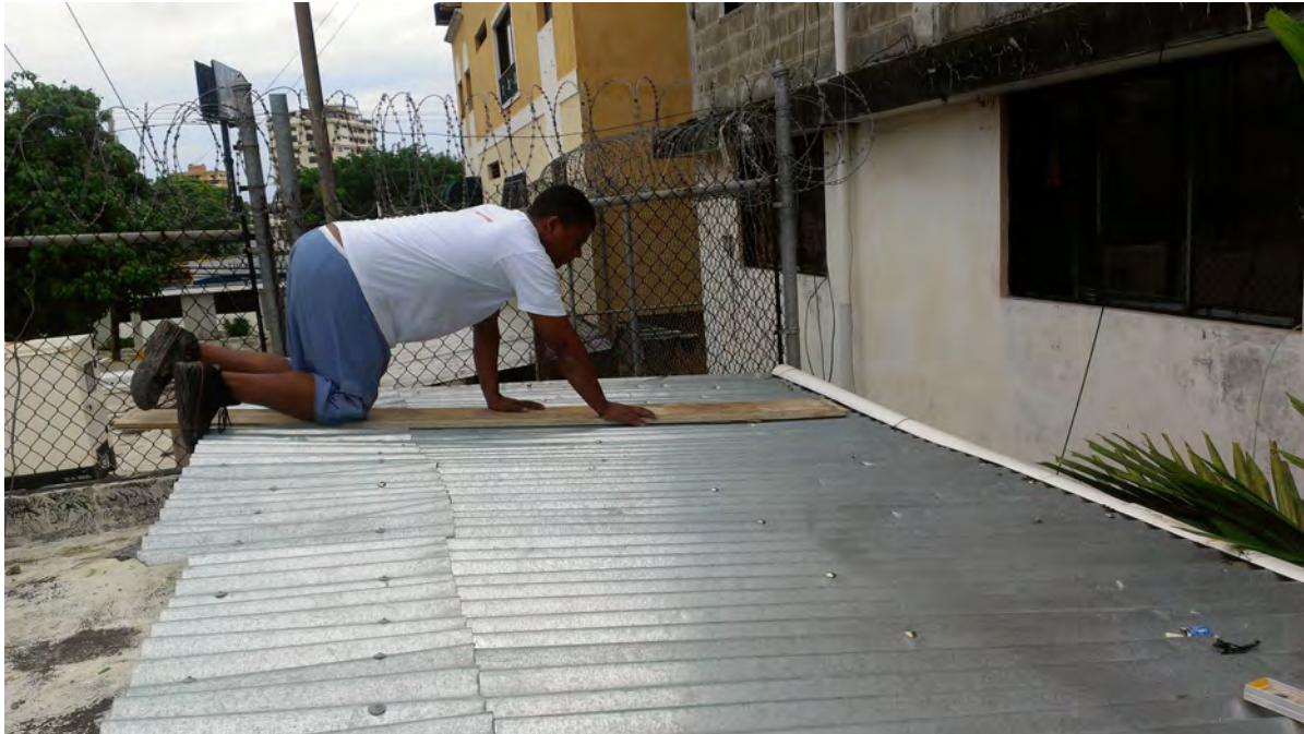
Figure 7.6: The community president works to improve the gutter by securing it to the roof with thicker wire.
