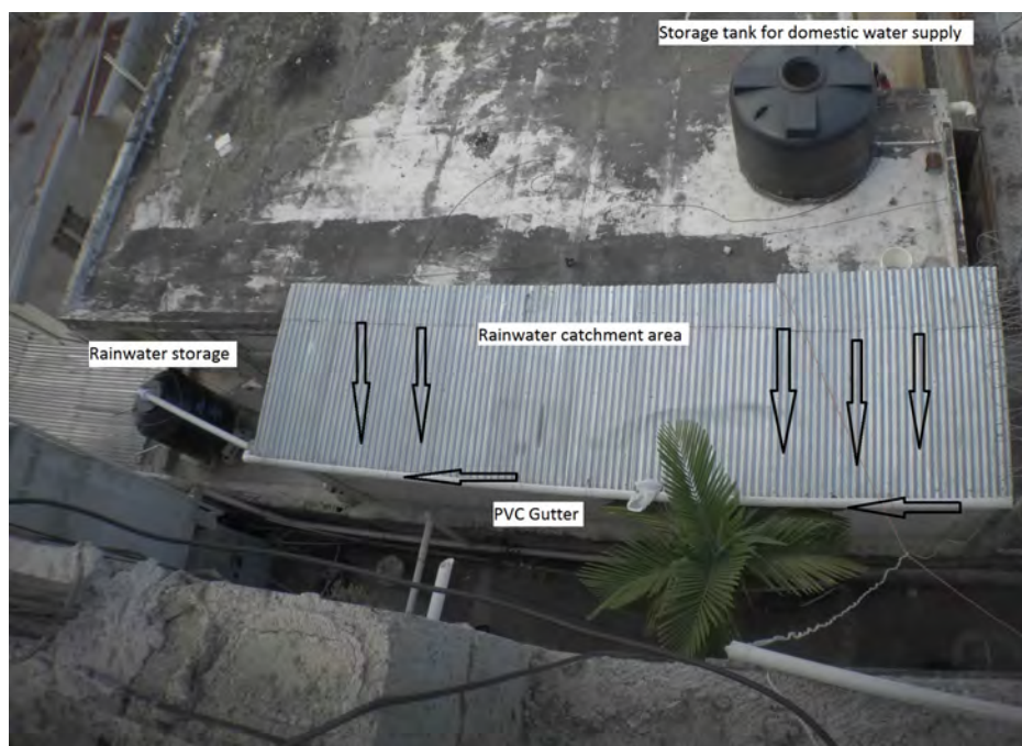
Figure 4.1: A view of the catchment area after some work by the 2012 rainwater team. Arrows indicate the flow direction of the captured runoff. Photo by Lonny Grafman.
