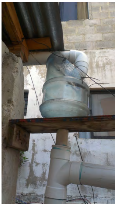
Figure 4.2: The primary screen separated leaves and other large particulate matter from the water flow. Screenings fell out of the way of the water flow by gravity. Beneath the primary screen was a Tee intersection, which directed water to the first flush system's storage pipes (below, partially pictured) and allowed water to enter the 250 gallon storage tank (right, not pictured).
