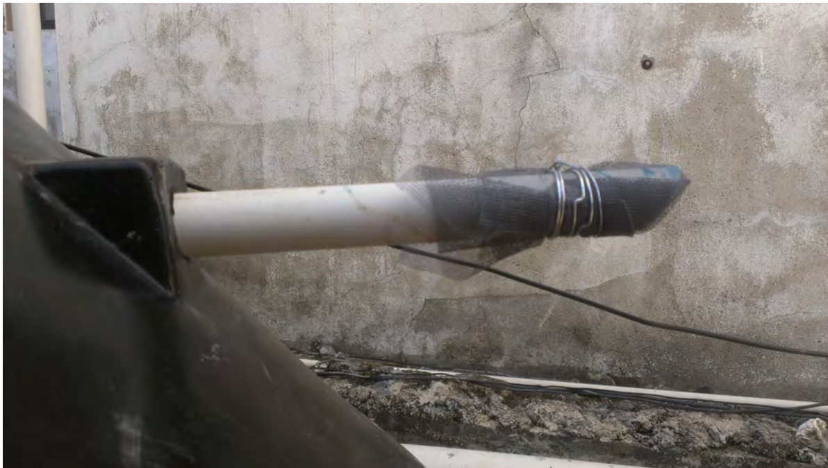
Figure 6.4: A short PVC pipe was attached to the overflow opening of the storage tank. The exposed end of the PVC pipe was cut at an angle and covered with plastic netting, secured by galvanized wire.
